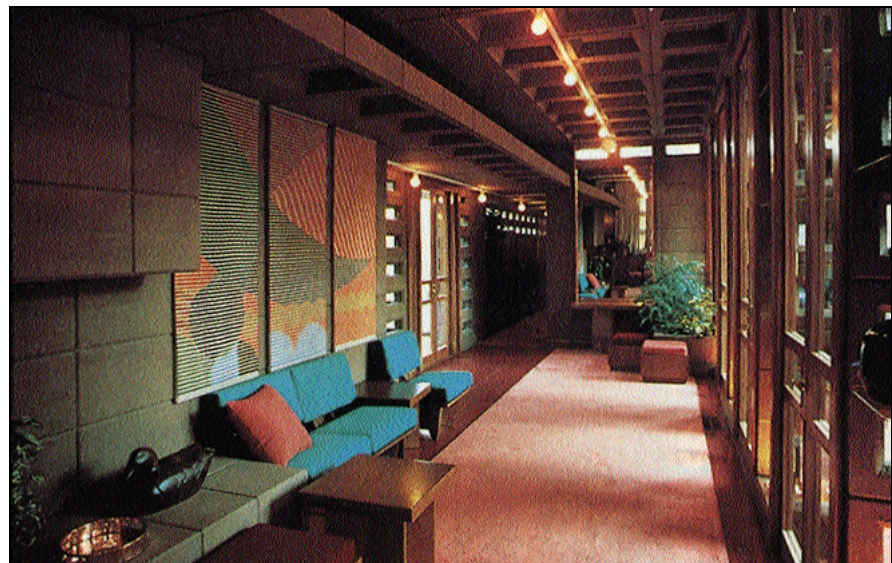
Interior view of the exhibit home shows deeply coffered concrete masonry ceiling. Window wall at the right is made up of concrete block units inset with glass. Note exposed standard Usonian Automatic blocks in the wall at the left.
